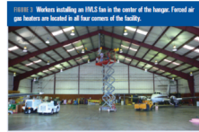
FIGURE 2 Workers installing an HVLS fan in the center of the hangar. Forced air gas heaters are located in all four corners of the facility.
